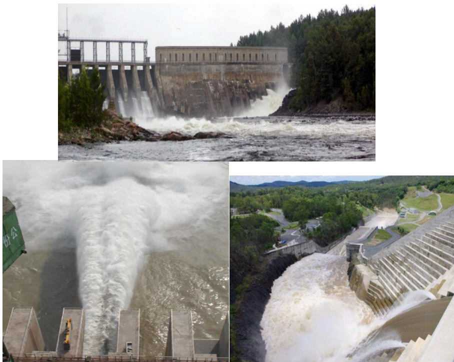
Fig. 1.1: Energy Dissipation in Hydraulic Structures
